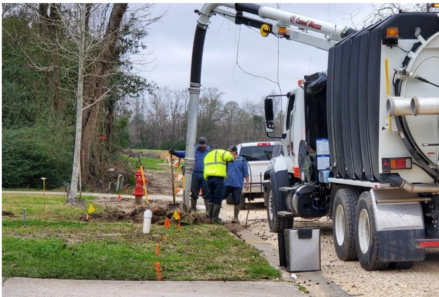
HOLLY ST. WATERLINE REPAIR HYDRO-EXCAVATION – JAYMES YOUNG, STEPHEN DAVILA AND NATHAN DAVID
