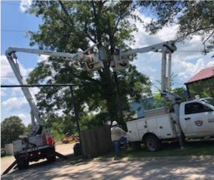
ELECTRICAL AERIAL WORK: CHARLES YPMA, CORY FORD AND COREY ROBINS
