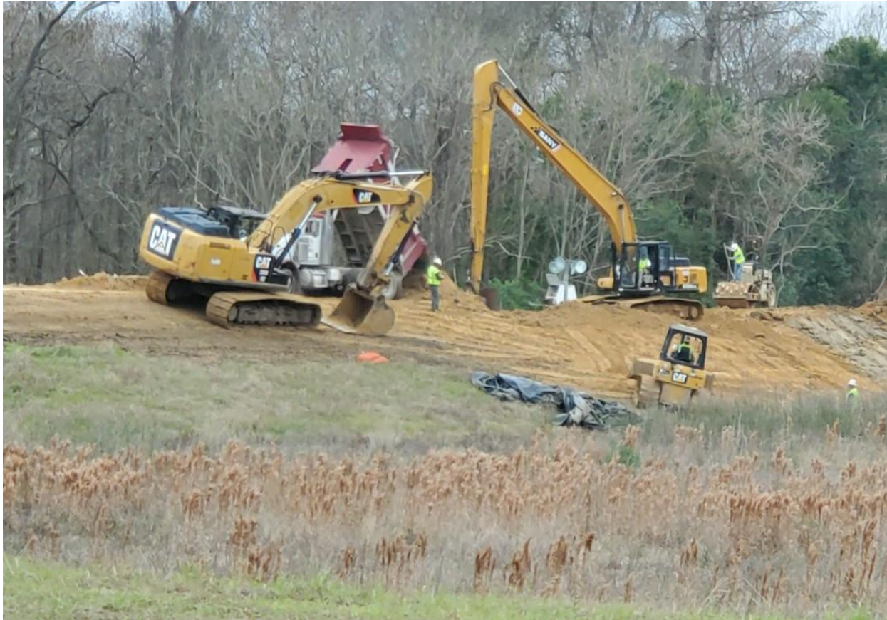
MAIN B LEVEE REPAIR – BACKFILL OF CULVERT SECTION
