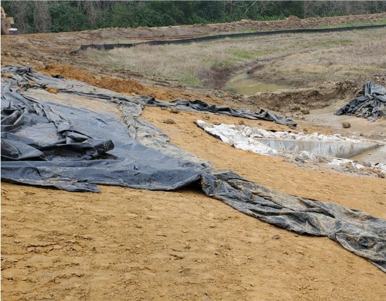
LEVEE INLET AND RIPRAP – INSPECTIONS BY JAMES REDDING
