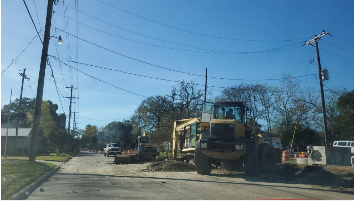
TEXAS STREET: STORM DRAINAGE INSTALLATION
