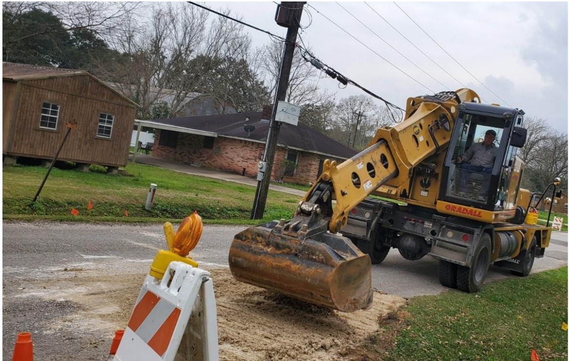
STREETS REPAIRING A SINKHOLE ON WASHINGTON ST. – RICK UBNOSKYE
