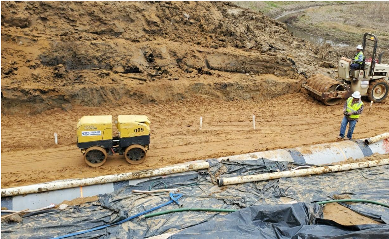
PLACING SELECT FILL IN THE CONCRETE PIPE SECTION OF THE LEVEE.
