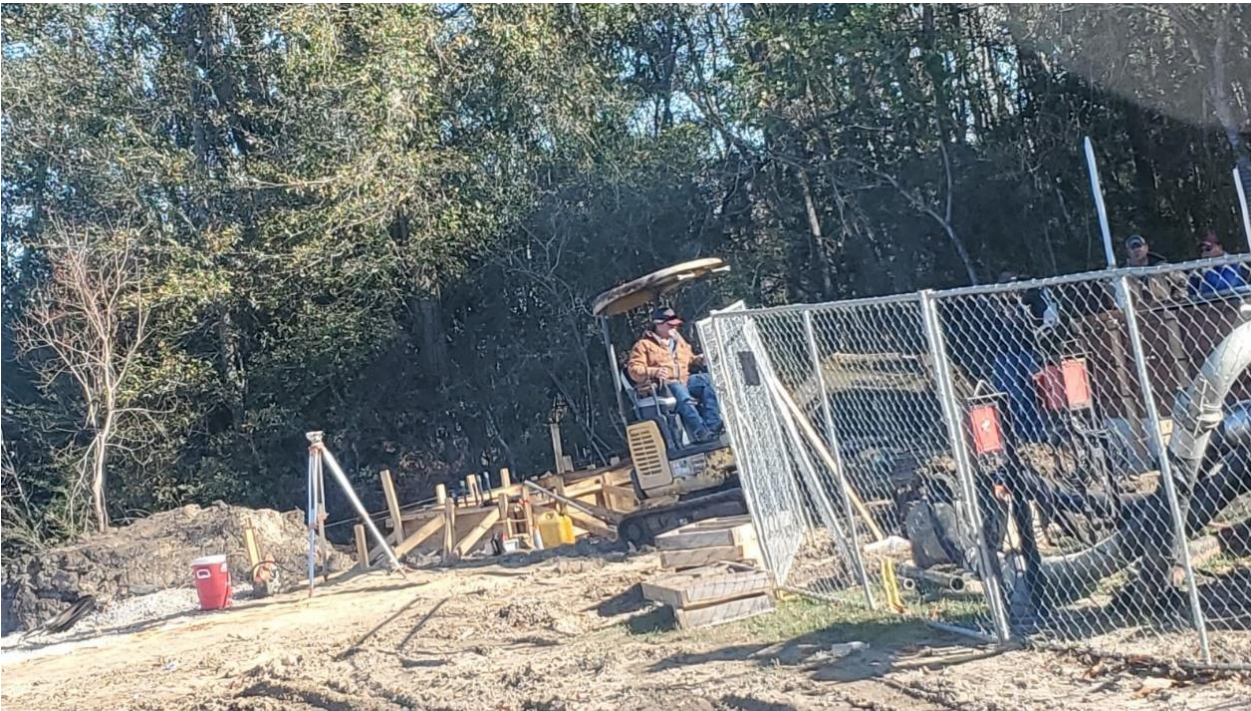
BEAUMONT LIFT STATION
