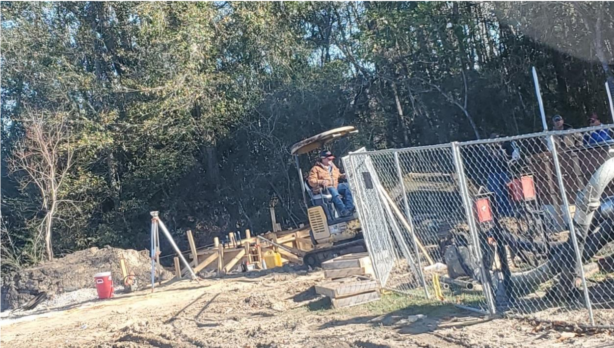
BEAUMONT LIFT STATION
