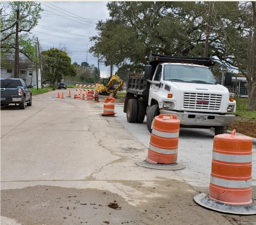
TEXAS ST. PAVEMENT REPAIRS
