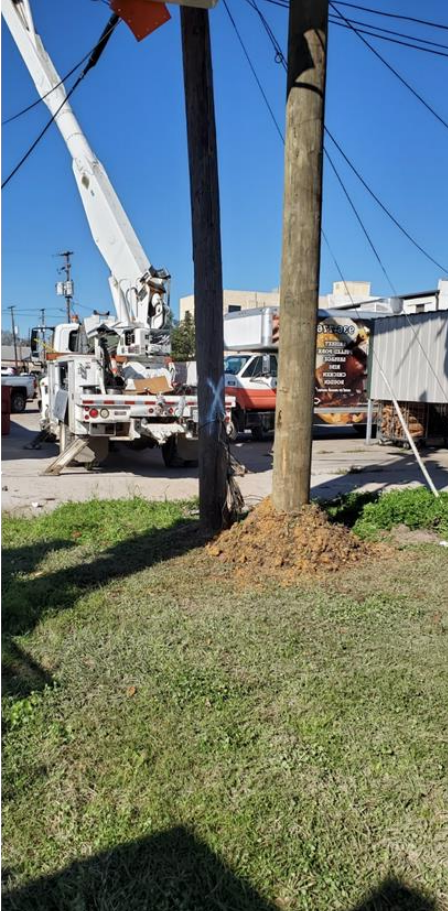
ELECTRICAL REPLACING POWER POLE MLK AND FANNIN ST.
