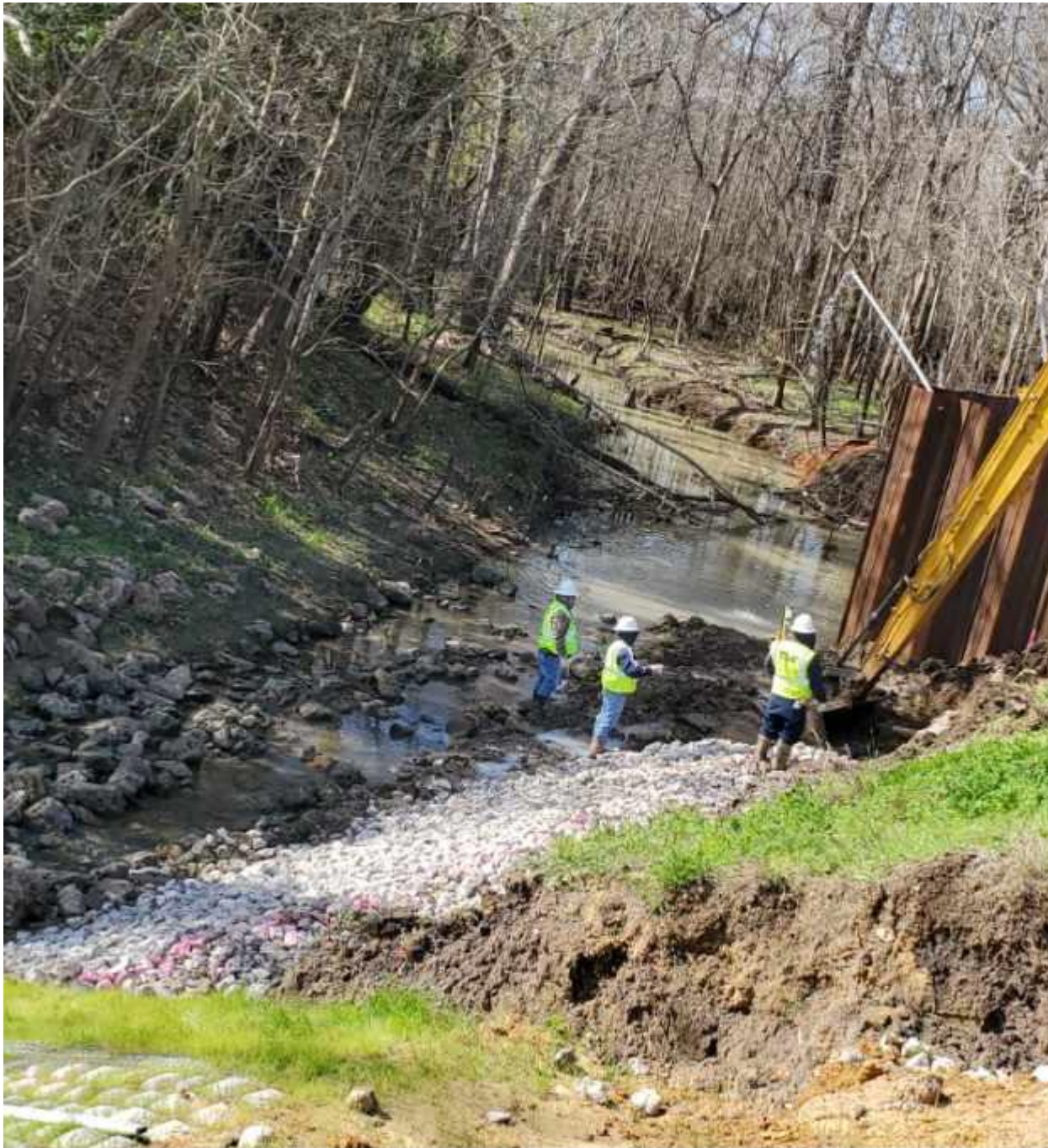
MAIN B LEVEE REPAIR – REMOVAL OF COFFER DAM
