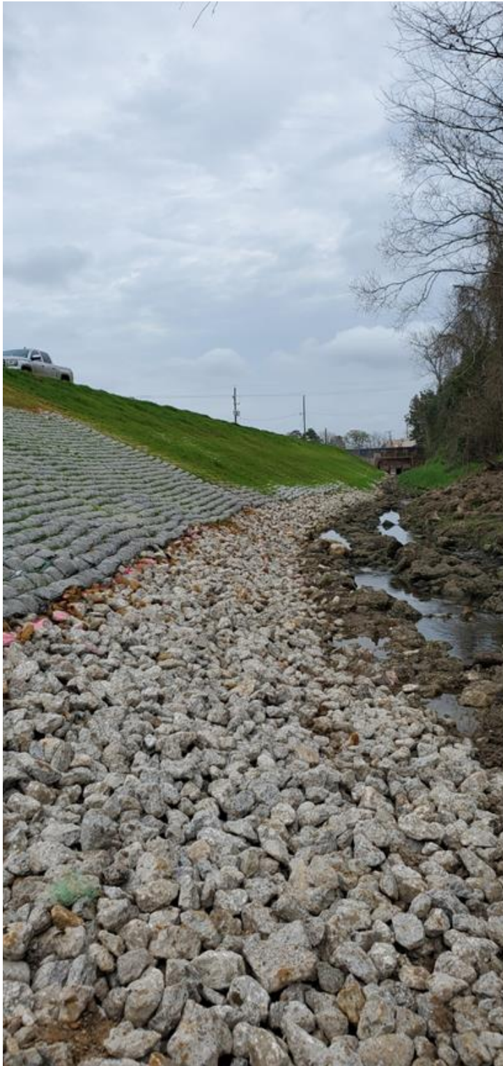
COMPLETED LEVEE SLOPE REPAIRS.
