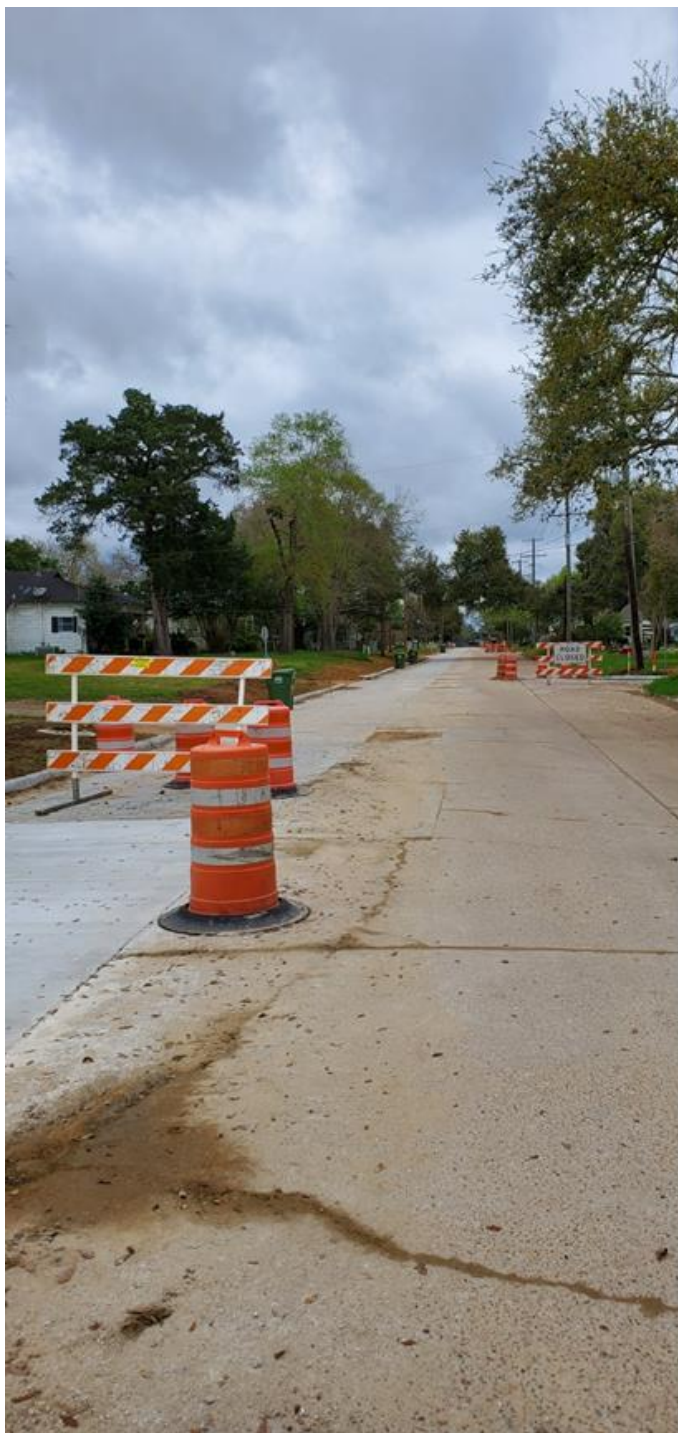
TEXAS STREET: PAVEMENT REPAIRS
