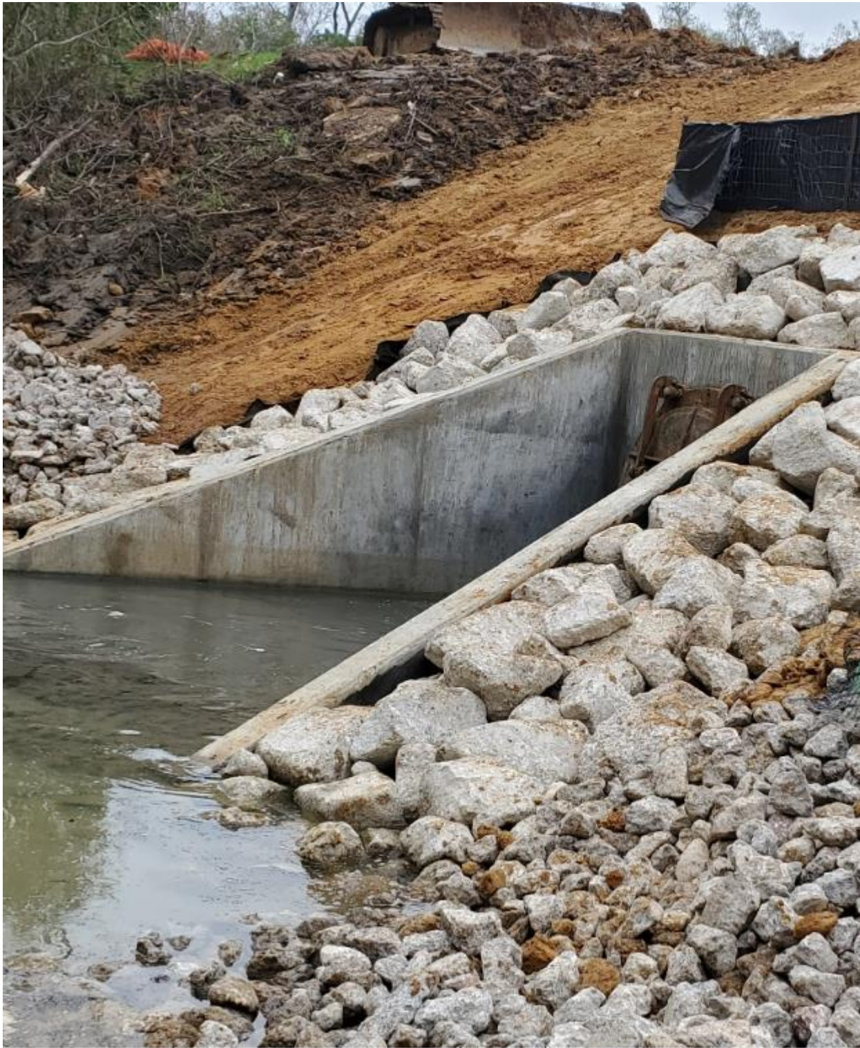
RIVERSIDE OUTLET WITH FLAPGATE AND RIPRAP – INSPECTIONS BY JAMES REDDING
