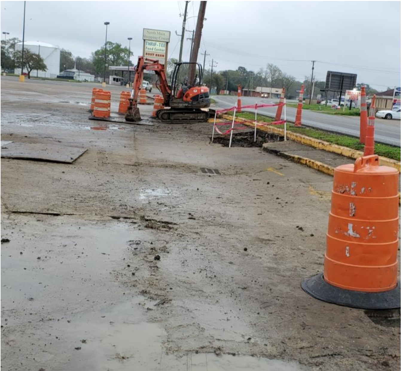
WATER LEAK REPAIR(6") UNDER THE MAIN ST. BOX CULVERTS NEAR BAYTOWN SEAFOOD
