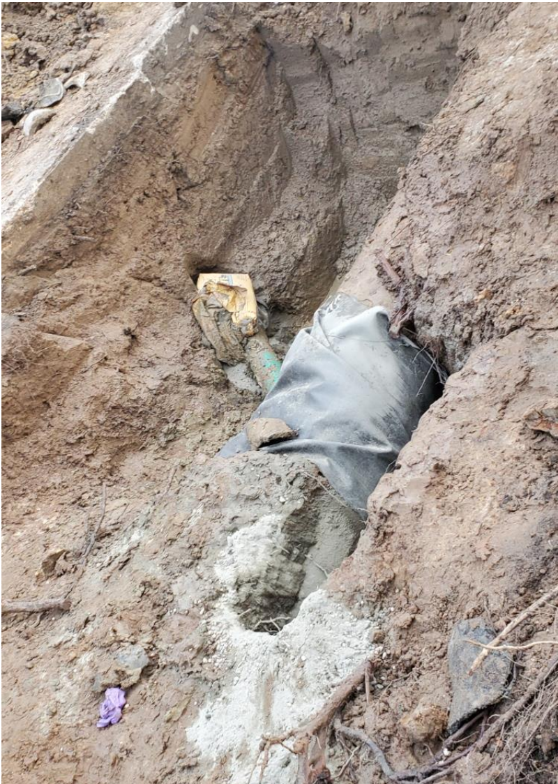
WASTEWATER REPAIR N. TRAVIS BETWEEN JEFFERSON AND HOLLY ST.
