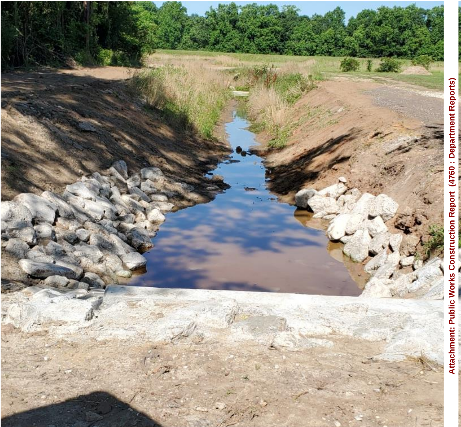
RIPRAP AT END OF HOLLY ST.
