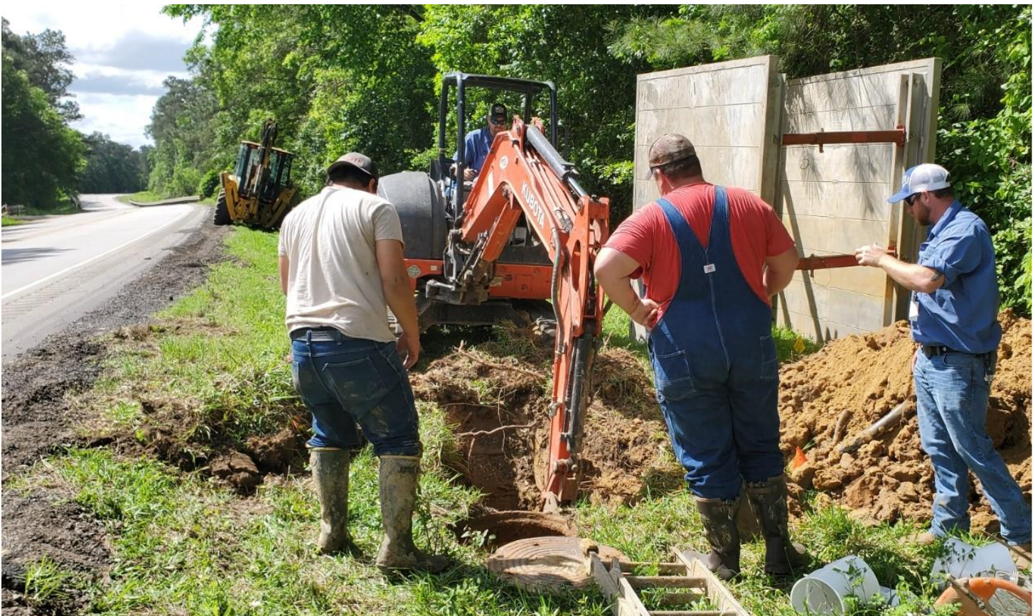
WASTEWATER INSTALLING A SANITARY SEWER TAP – STEPEN DAVILLA, DALE PITTS AND CHAD CALLAWAY.
