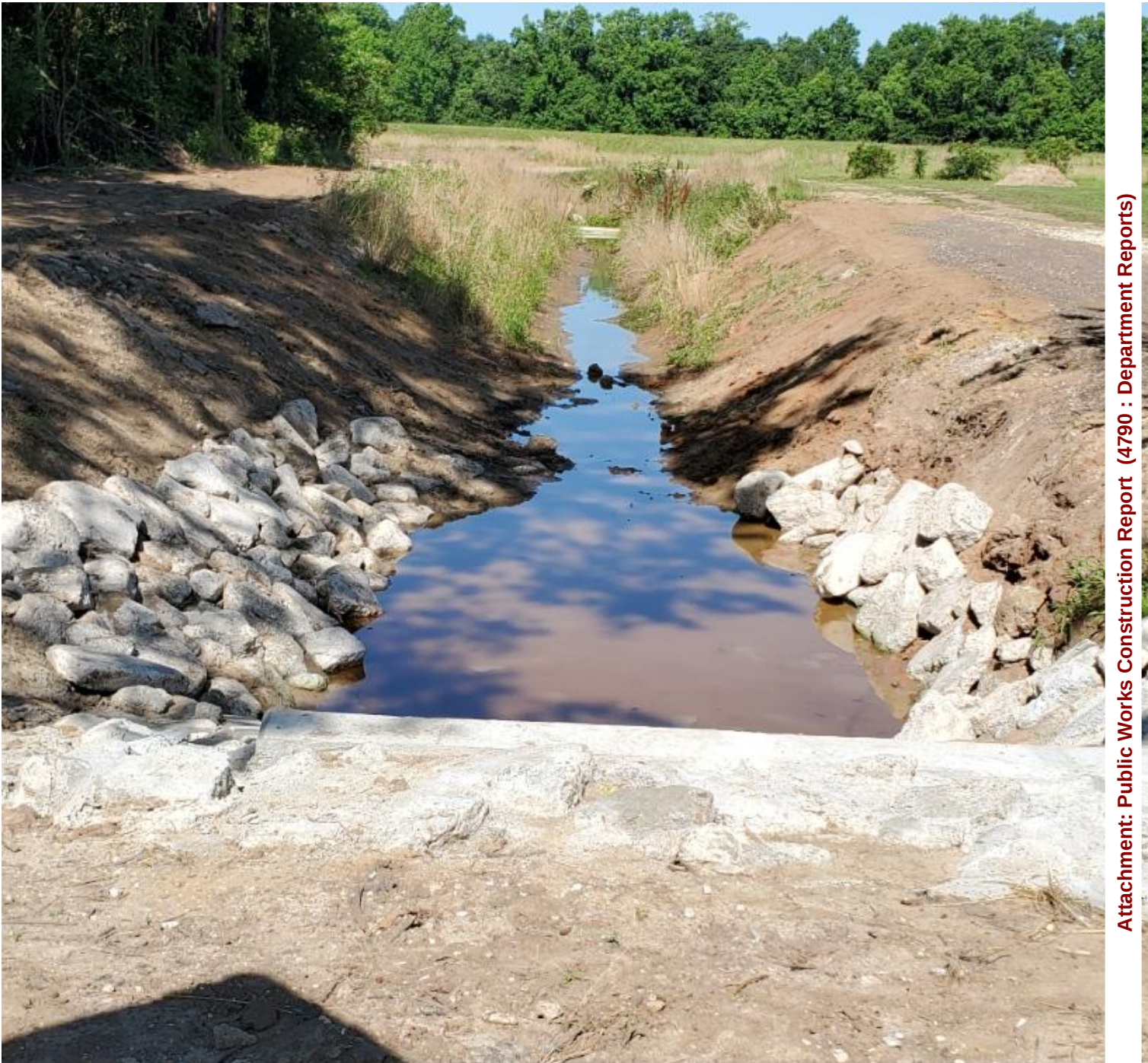
RIPRAP AT END OF HOLLY ST.
