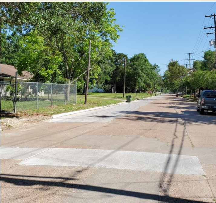
TEXAS ST. PAVEMENT REPAIRS
