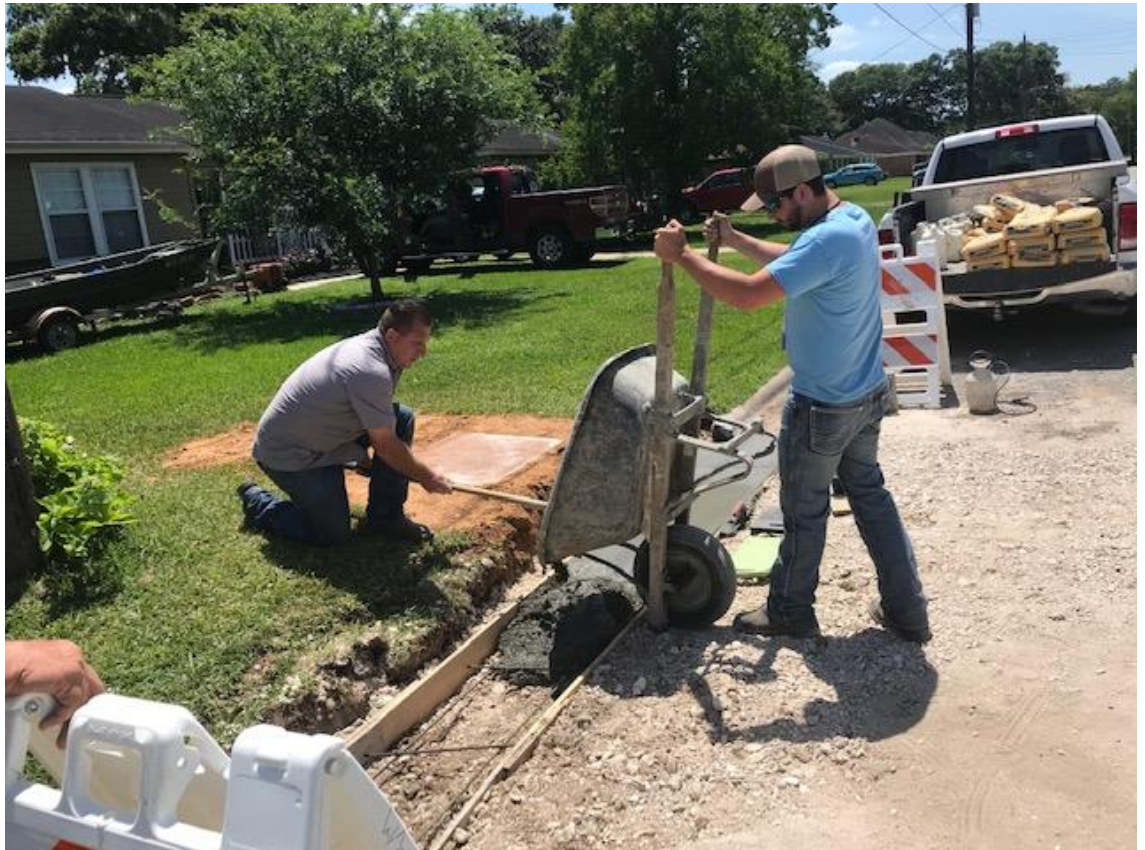
STREETS REPAIRING CURB AND GUTTER AFTER REPAIRING A SINK HOLE – PATRICK MITCHUM, JAMIE RODABAUGH
