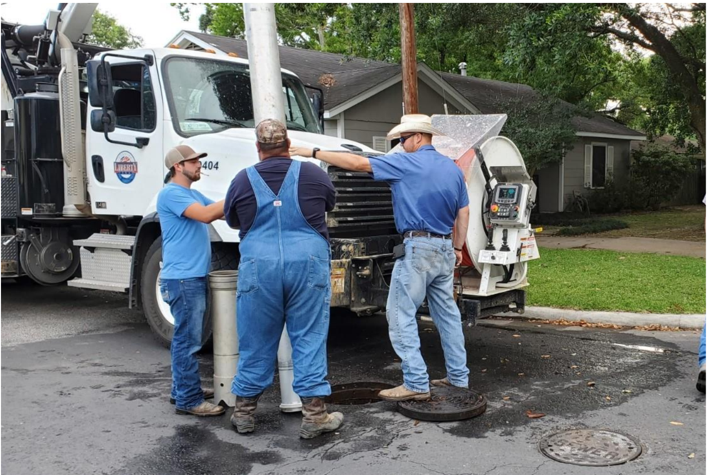
EDGEWOOD ST. - WATER CREW HELPING STREETS CLEAR A STORM SEWER AHEAD OF A THUNDERSTORM – DAVID ALLISON, CHAD CALLAWAY, PATRICK MITCHUM AND RAYMOND KOCIAN
