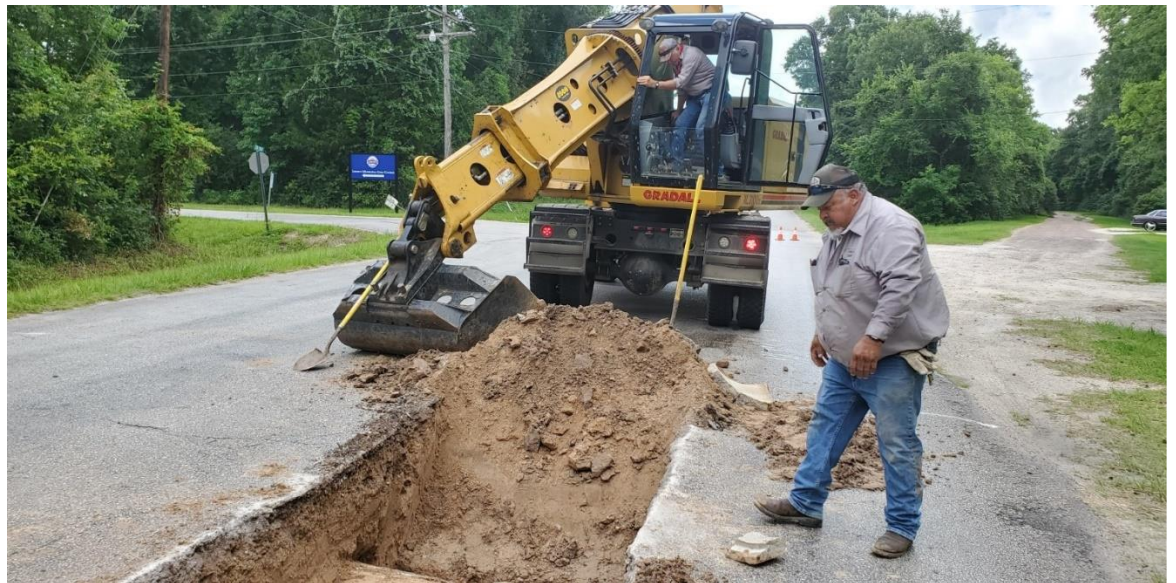
STREETS REPAIRING STORM SEWER CULVERT ON BEAUMONT AVE. NEAR THE MUNICIPAL GOLF COURSE – JESSE VARA AND RICK UBNOSKYE
