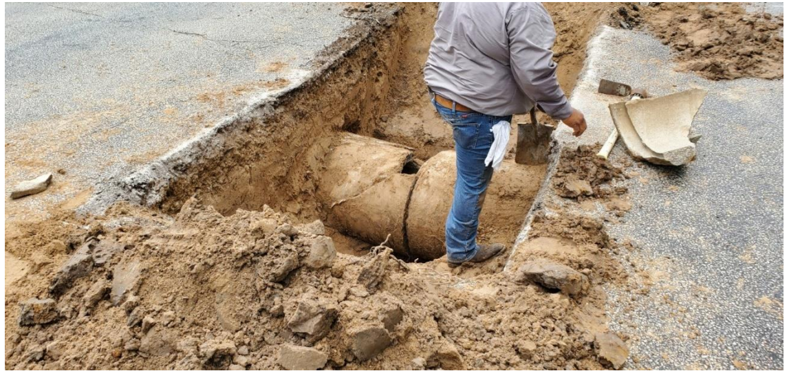
STREETS REPAIRING STORM SEWER CULVERT ON BEAUMONT AVE. NEAR THE MUNICIPAL GOLF COURSE – JESSE VARA
