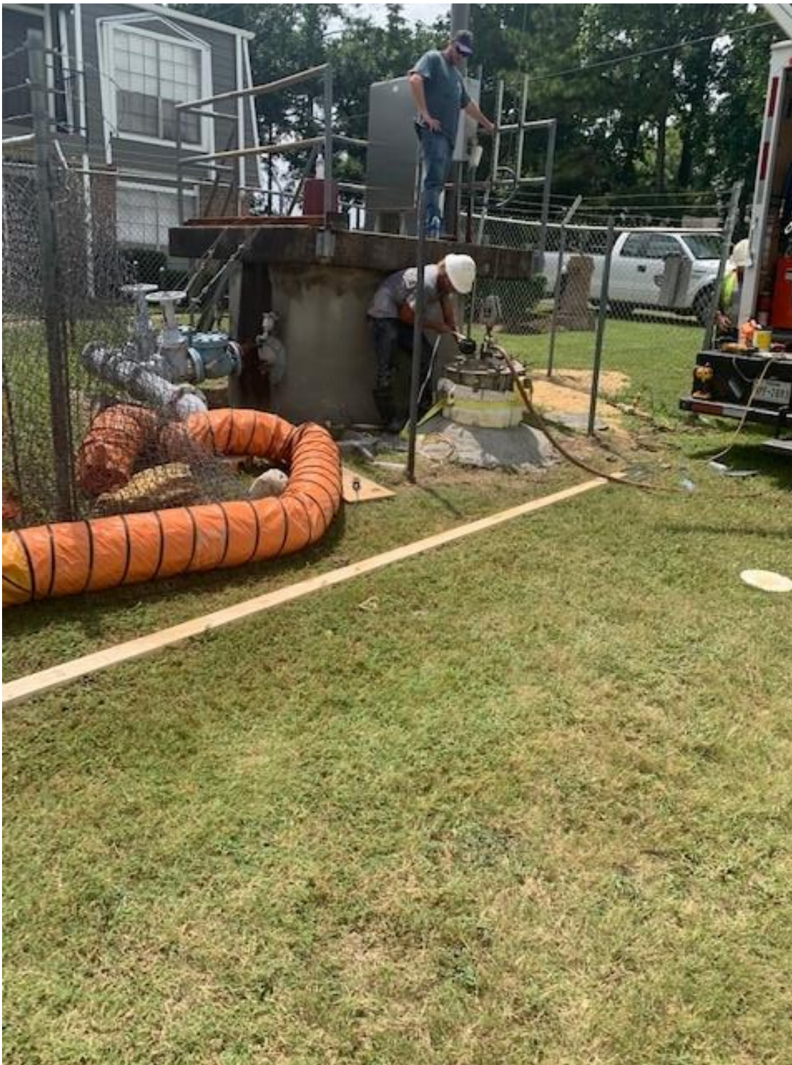
MANHOLE REHABILITATION-TRAVIS LIFT STATION
