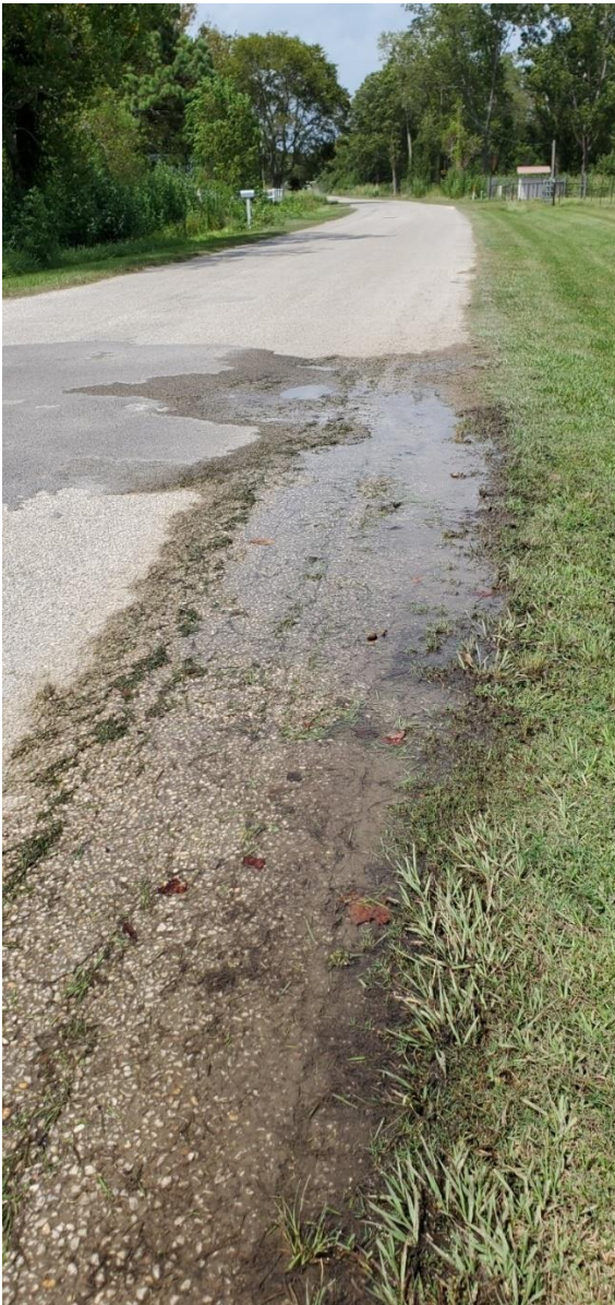
WATERLEAK INVESTIGATED ON OILFIELD RD.
