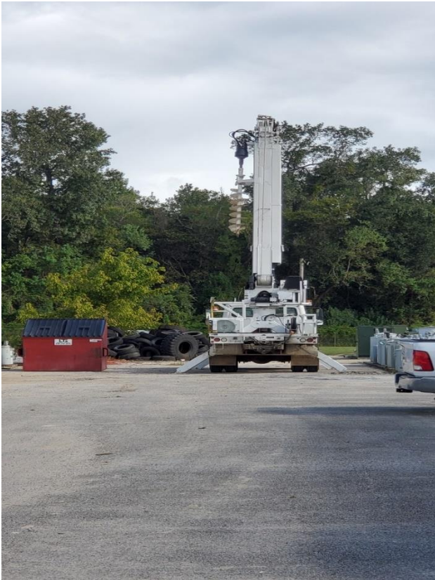
ELECTRICAL DEPARTMENT ORGANIZING TRANSFORMERS
