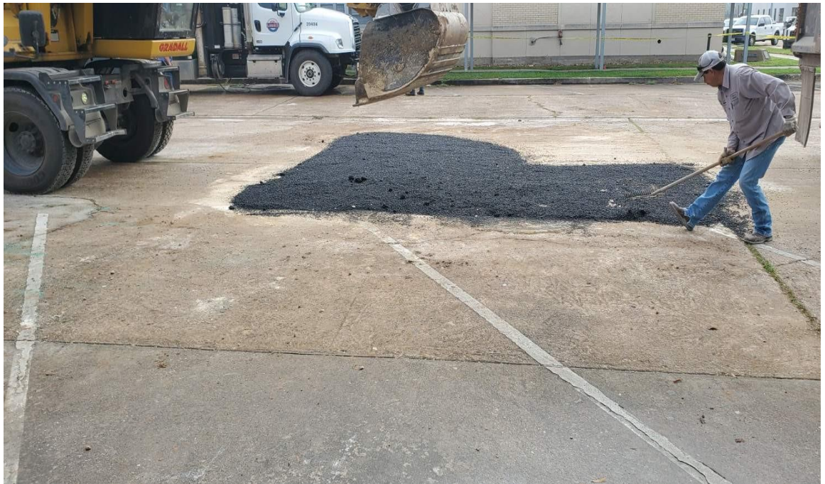
STREETS REPAIRING CAVITY UNDER TRINITY IN FRONT OF CITY HALL, VICTOR RACKING ASPHALT.
