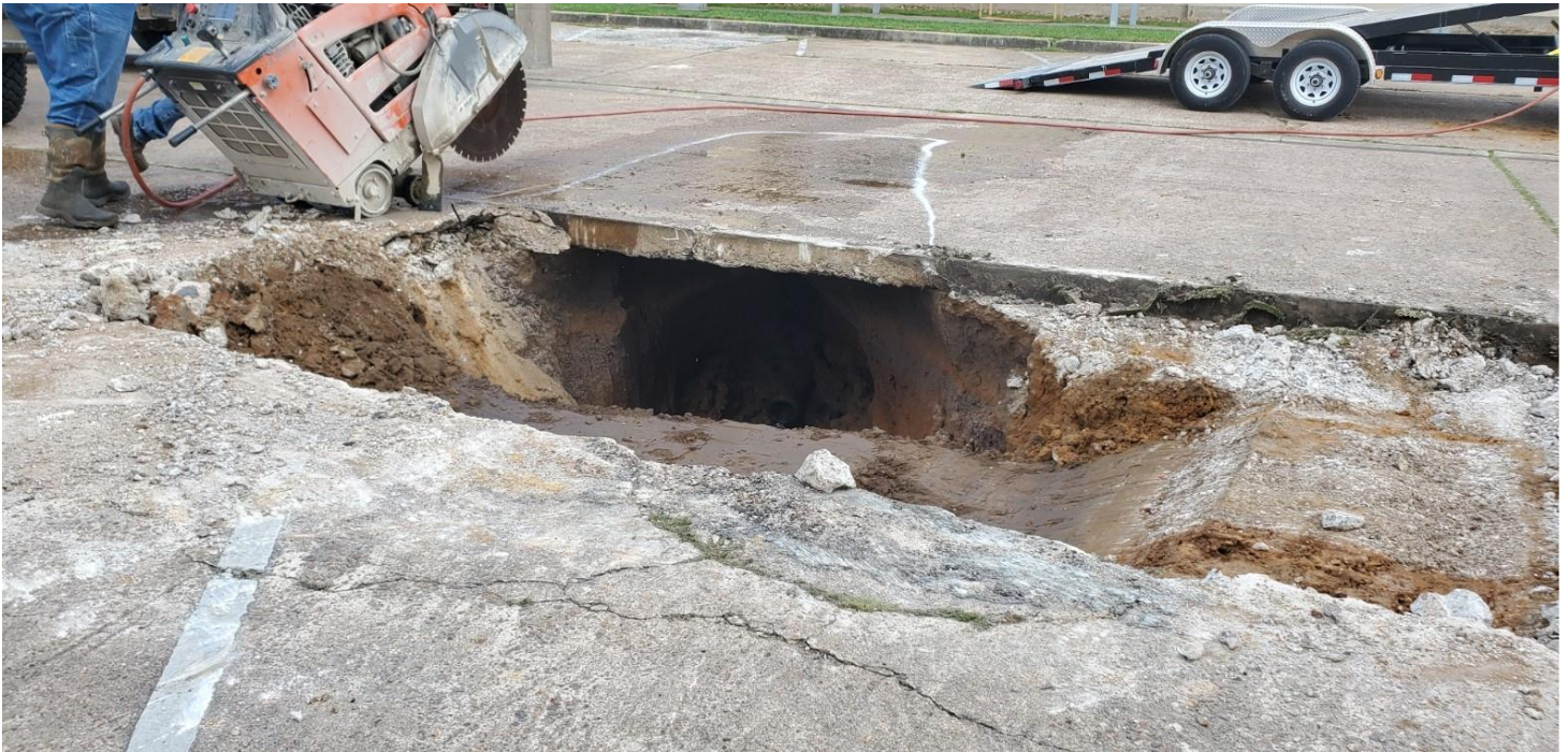
SANITARY SEWER CAVITY UNDER TRINITY ST. IN FRONT OF CITY HALL, WATER DEPARTMENT CUTTING PAVEMENT.
