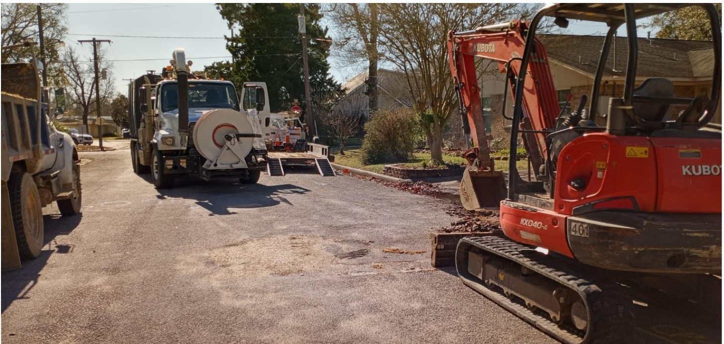
WATER DEPARTMENT REPAIRING A WATER LEAK AT COLUMBIA ST.
