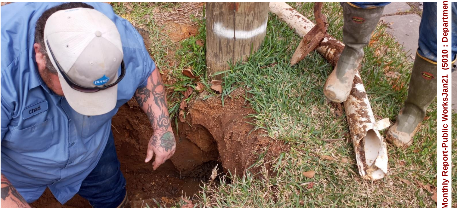
WATER DEPARTMENT REPAIRING A SANITARY SEWERLINE AT COLUMBIA ST. – CHAD CALLAWAY
