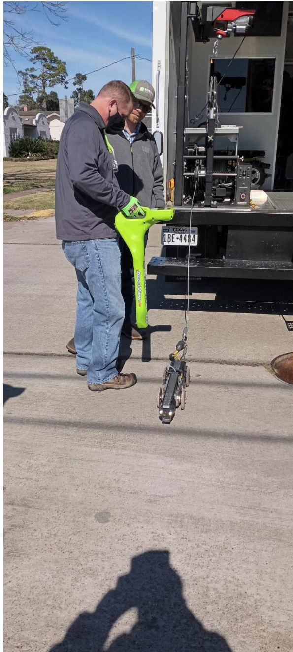
DEMONSTRATION OF SEWER PIPE INVESTIGATIVE EQUIPMENT
