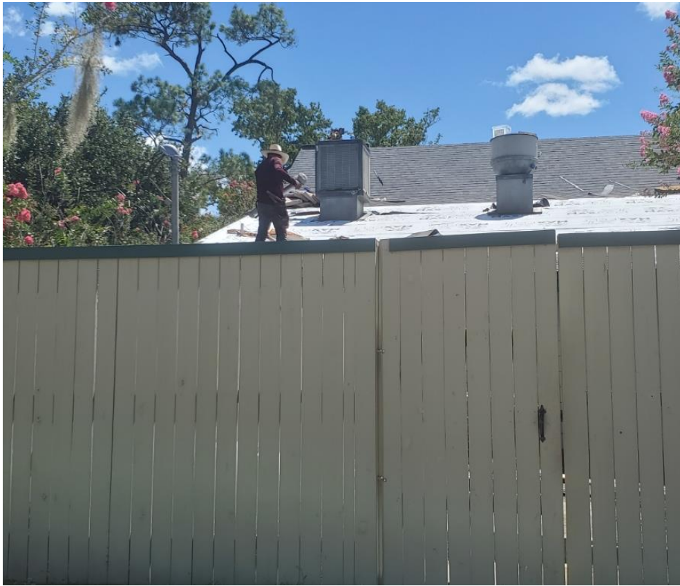
Contractors replacing roof on clubhouse
