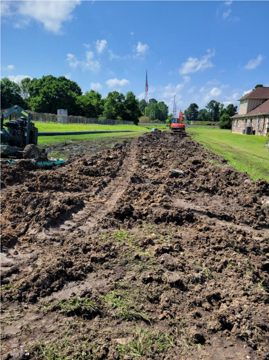
INSTALLATION OF 16" SEWER LINE ON BEAUMONT ST
