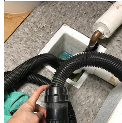
Cleaning out an AC drain line.
