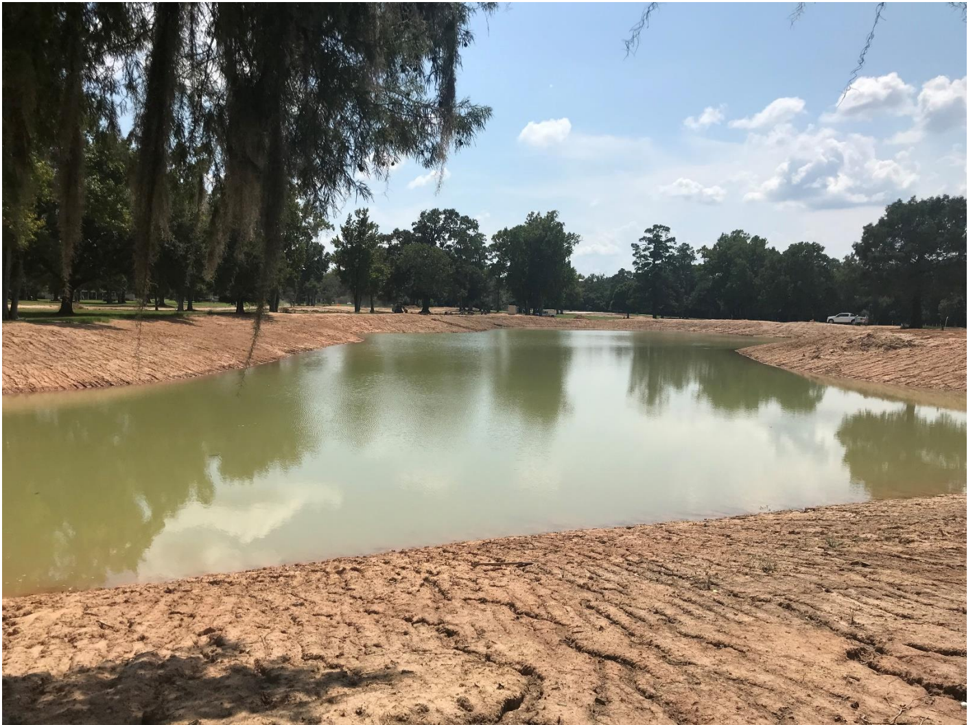
Irrigation lake being filled with water
