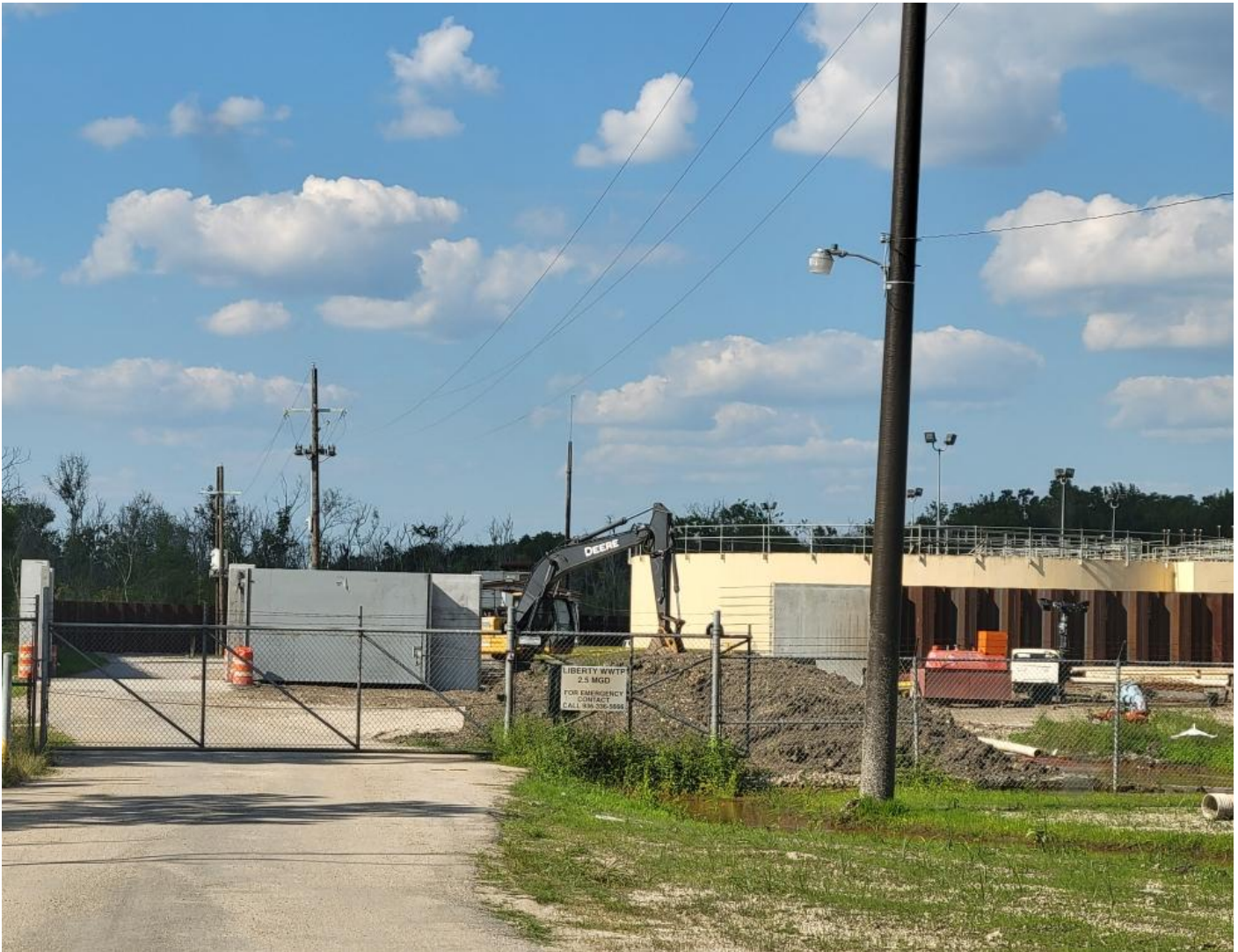
SHEET PILING ALONG THE FRONT OF THE WW TREATMENT PLANT. FLOOD GATE BEING INSTALLED
