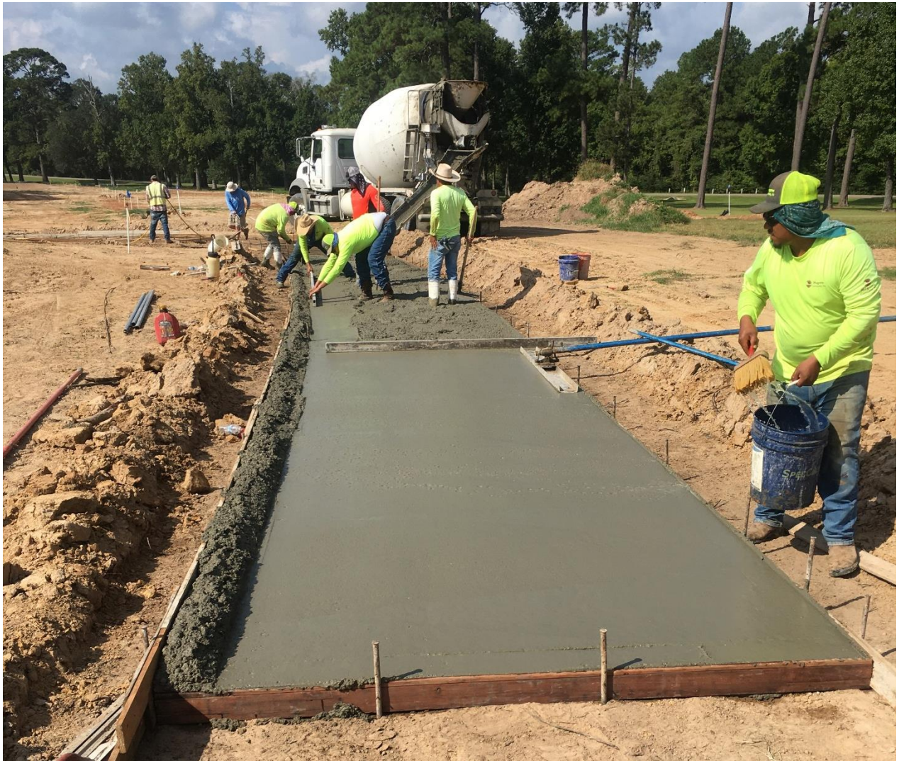
Contractors pouring concrete cart paths
