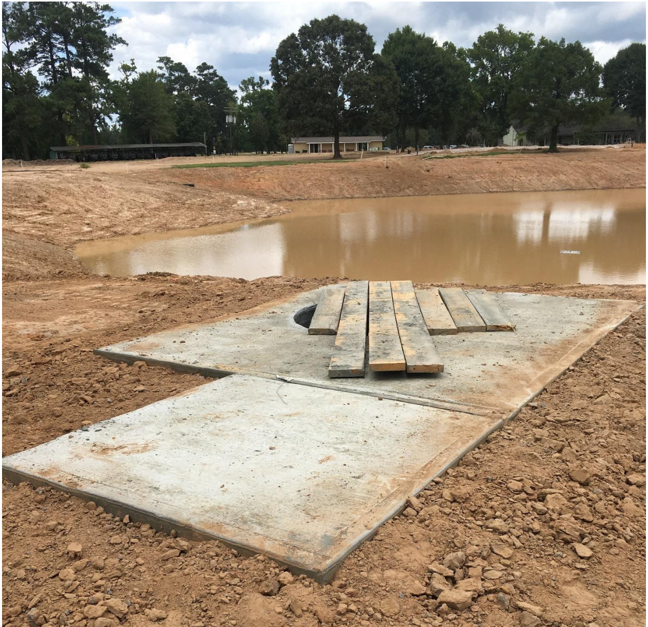
New pump station pad
