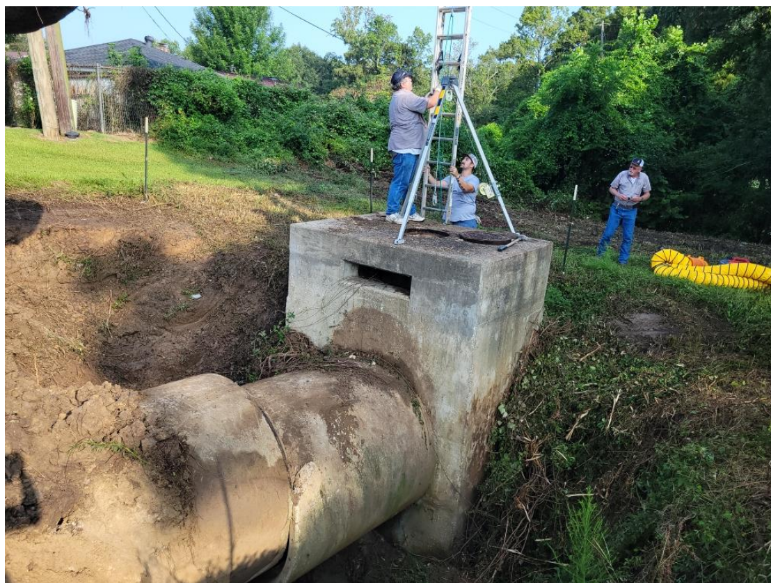
Forest Hills Storm sewer separation: Arthur, Brandon and Raymond
