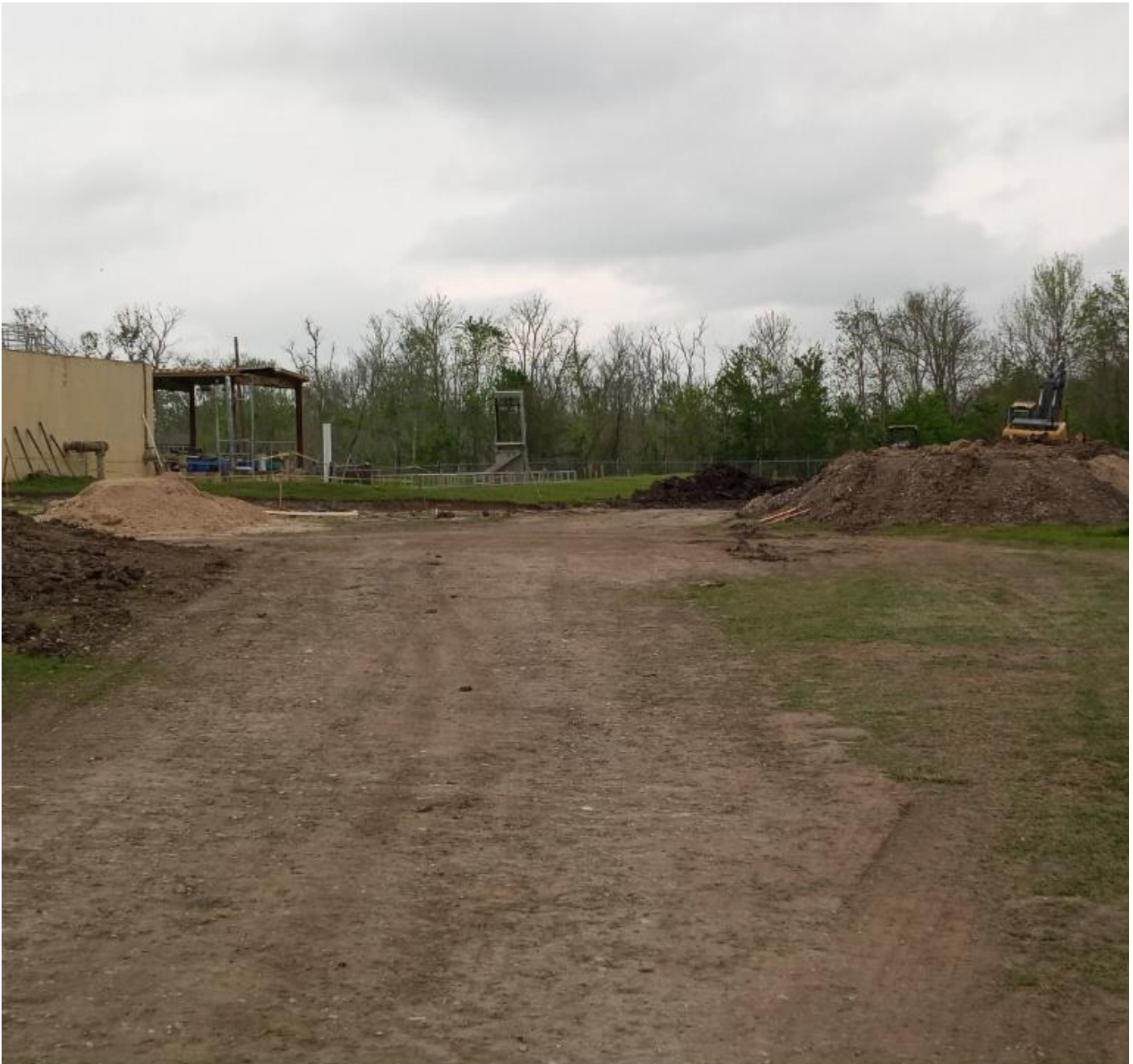
This is looking towards the rear of the Wastewater Treatment Plant.
