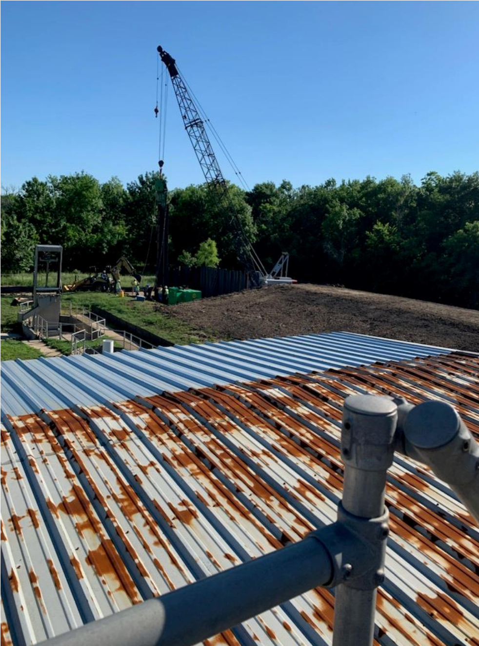
EARTHEN BERM BEHIND THE WW TREATMENT PLANT
