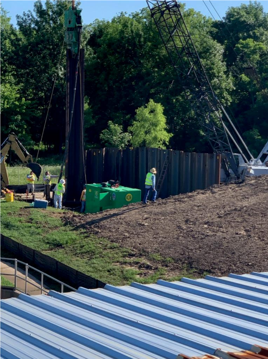
SHEET PILING IN THE BACK OF THE WW TREATMENT PLANT
