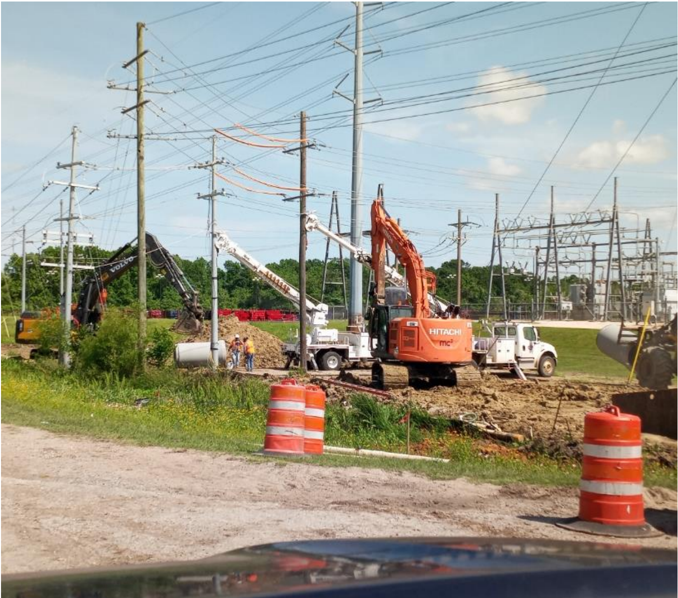
OUTFALL INSTALLATION UNDER POWERLINE CONFLICT ON FM 3361
