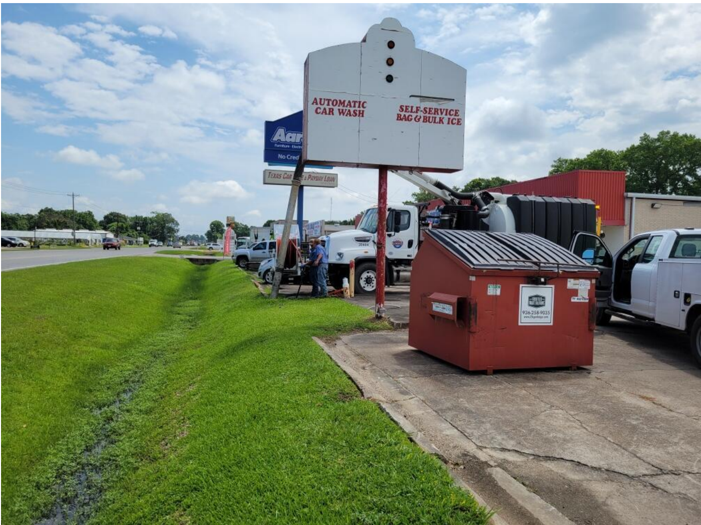
SANITARY SEWER MAINTENANCE ON N. MAIN ST.
