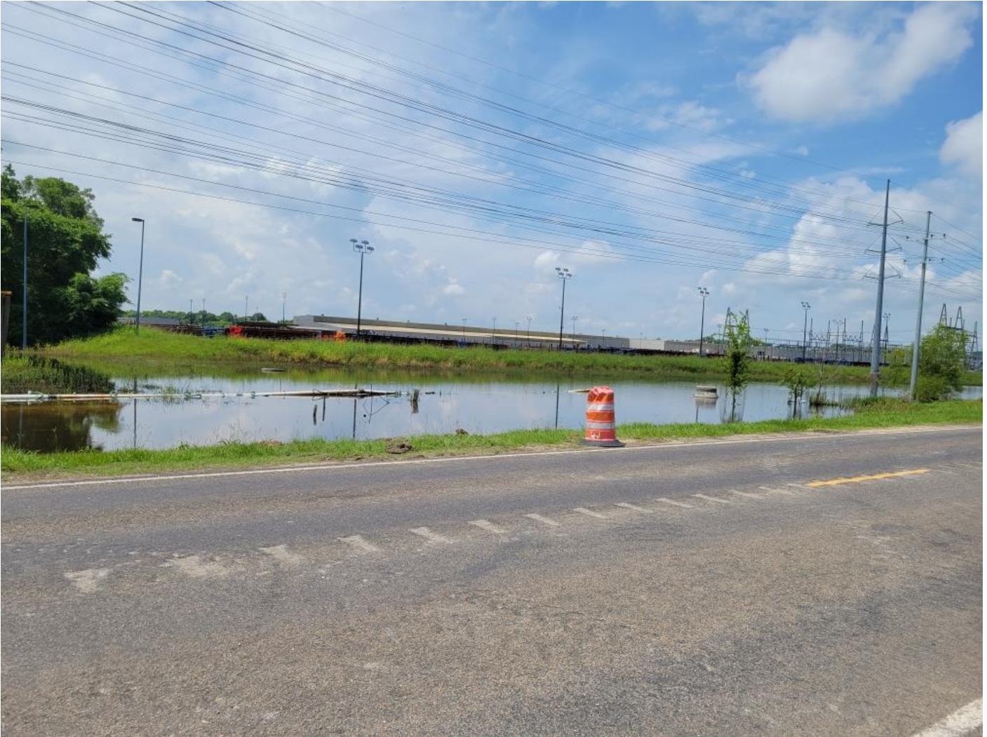
OUTFALL INSTALLATION UNDER WATER ON FM 3361
