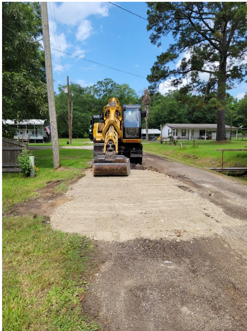
BASE REPAIRS ON AVENUE E
