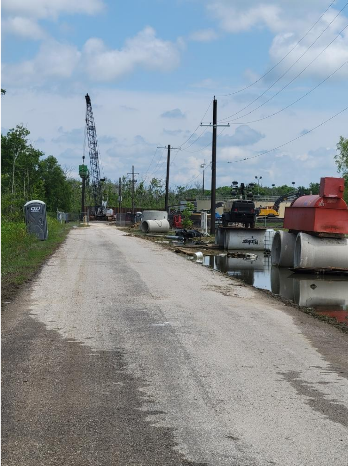
SHEET PILING ALONG BACK AND SIDE OF THE WW TREATMENT PLANT
