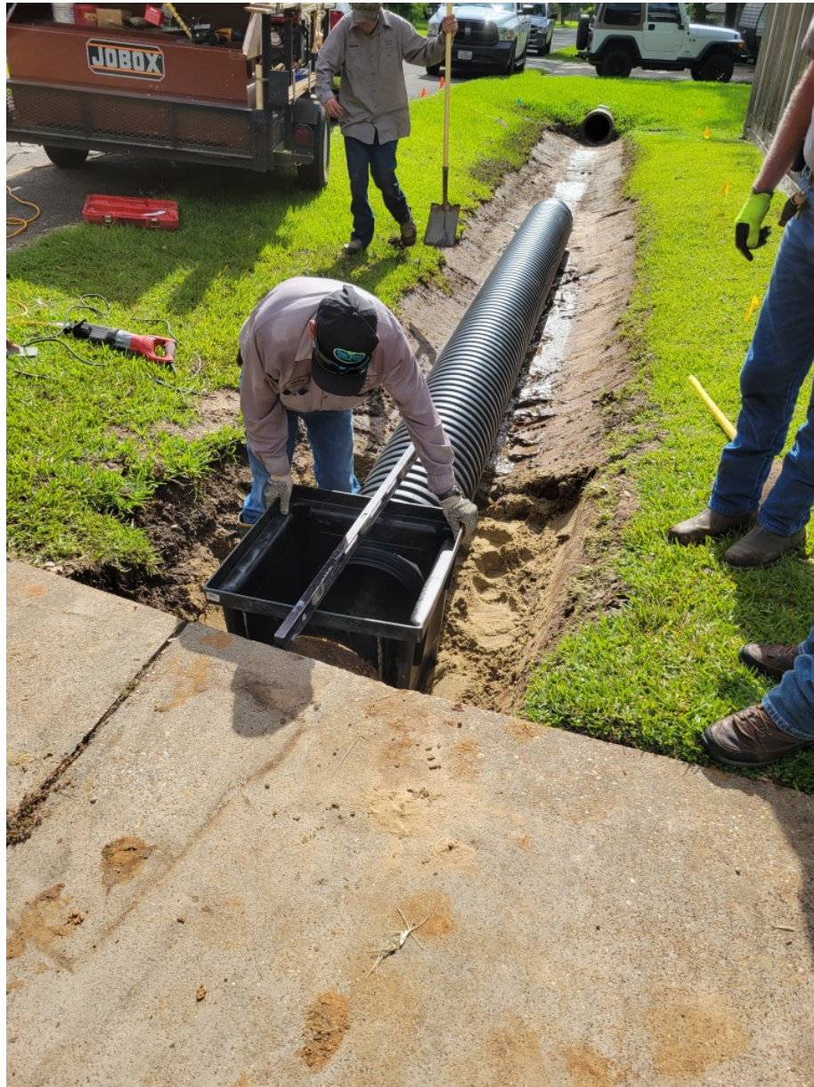
Installing driveway culvert on Star Ridge St.; Victor, Rick, Nathan
