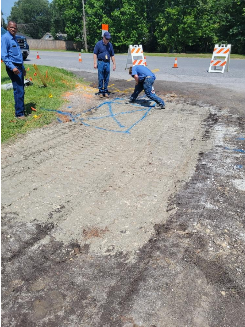
Minglewood and HWY 146 completed; Mark Reed, Wayne, Robert
