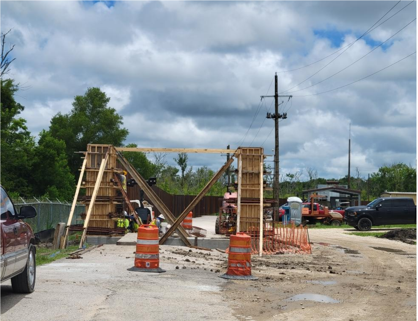
WW TREATMENT PLANT FLOODGATE CONSTRUCTION AT THE ENTRANCE
