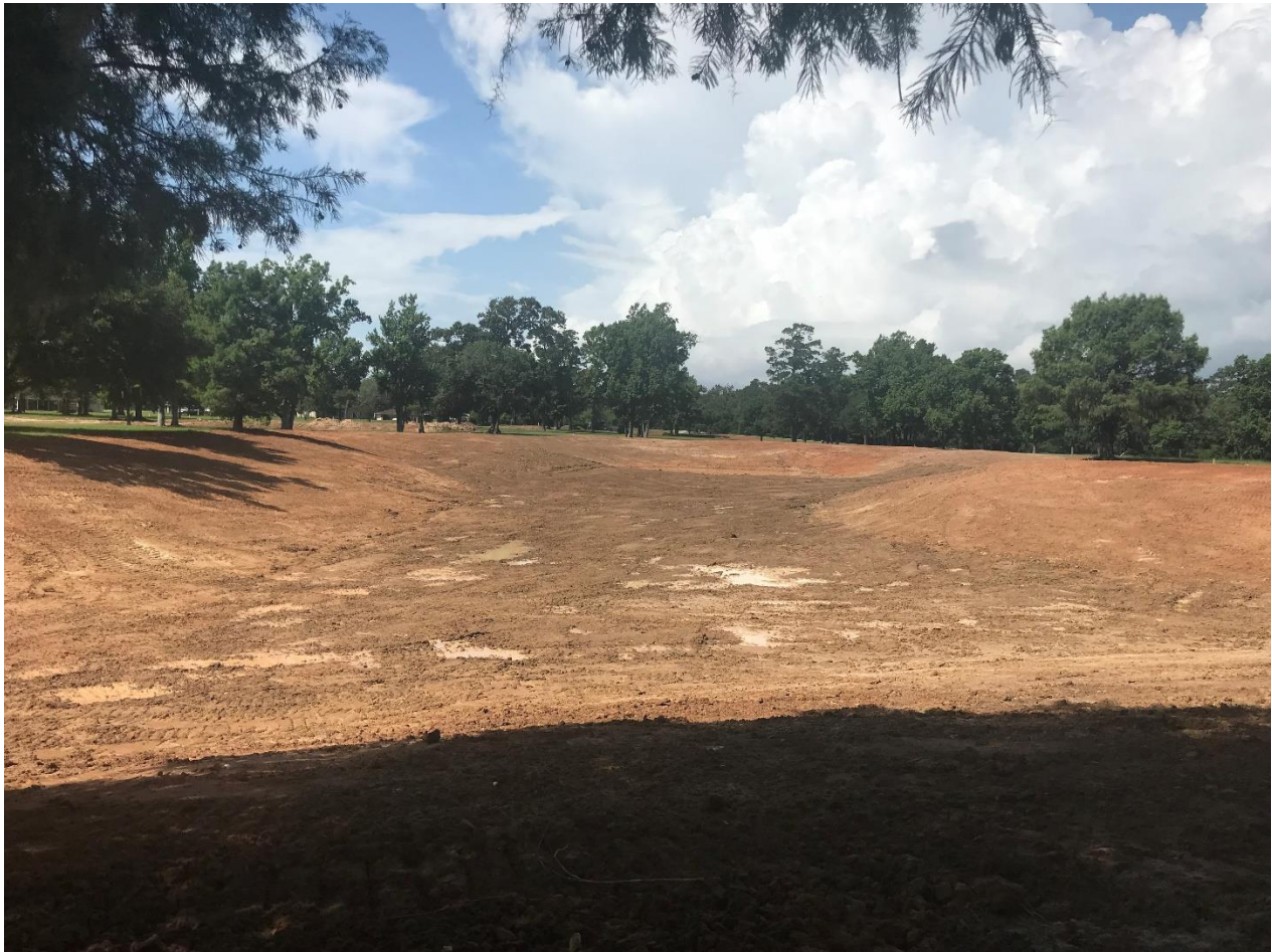
Completed irrigation lake
