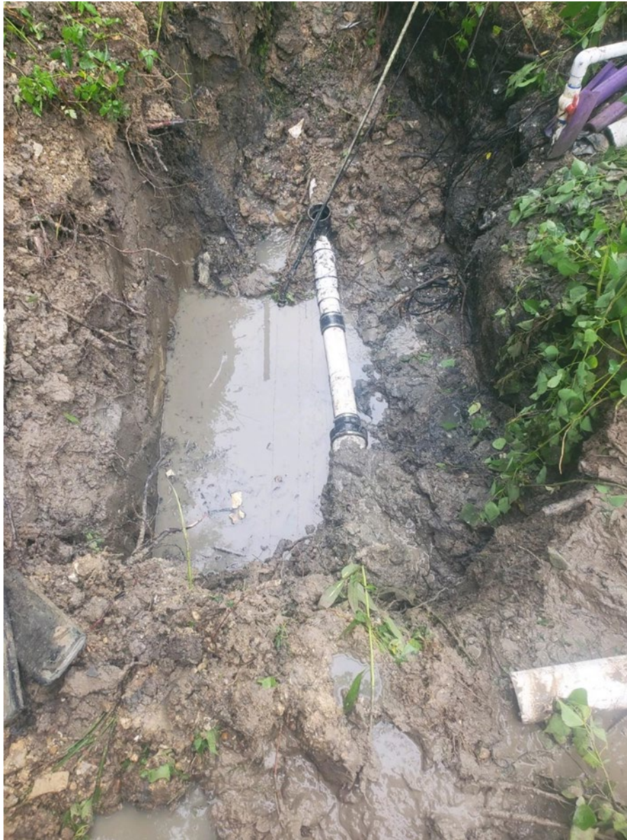
Sanitary sewer replacement Beaumont St.
