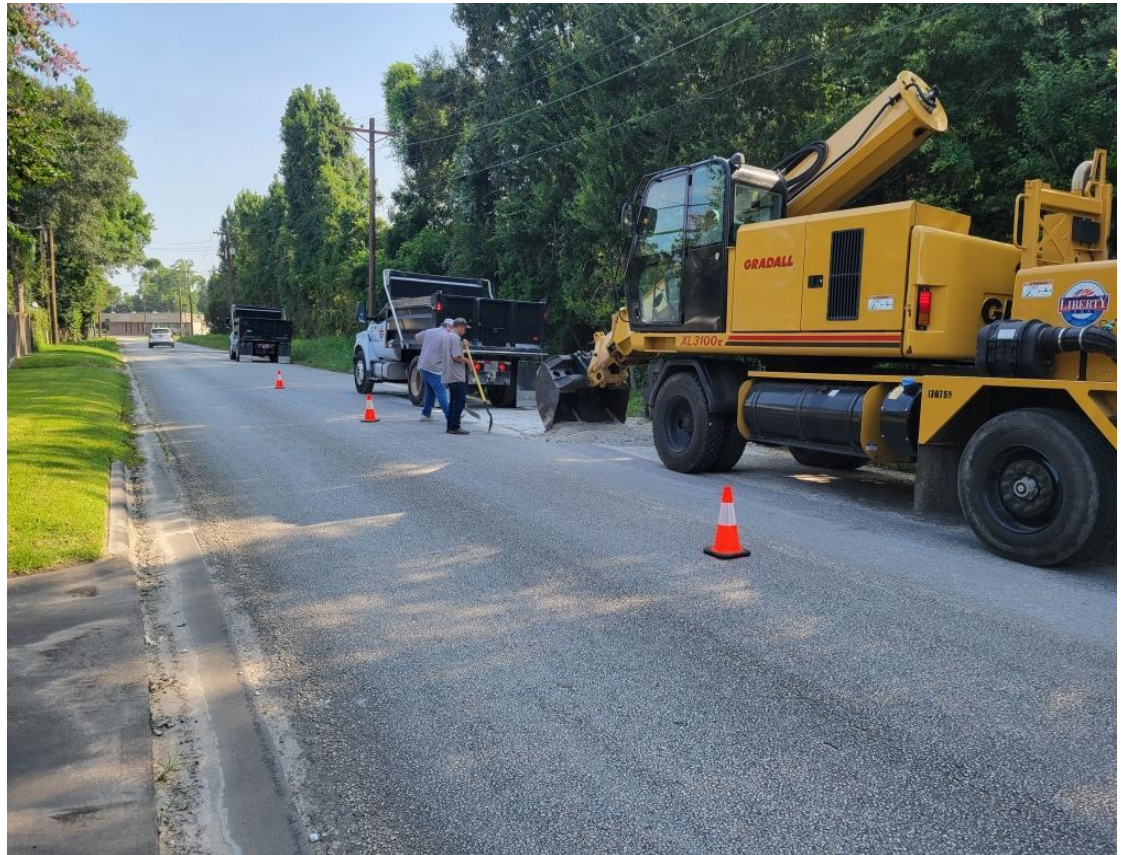
Full depth street repairs on Texas St. Rick, Nathan and Arthur
