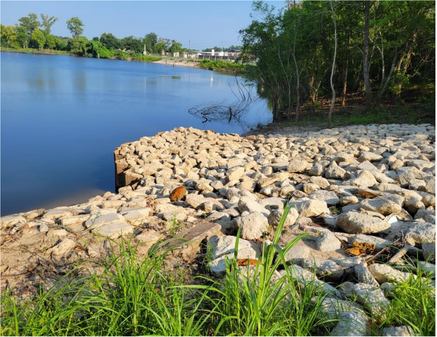
WW TREATMENT OUTFALL BULKHEAD
