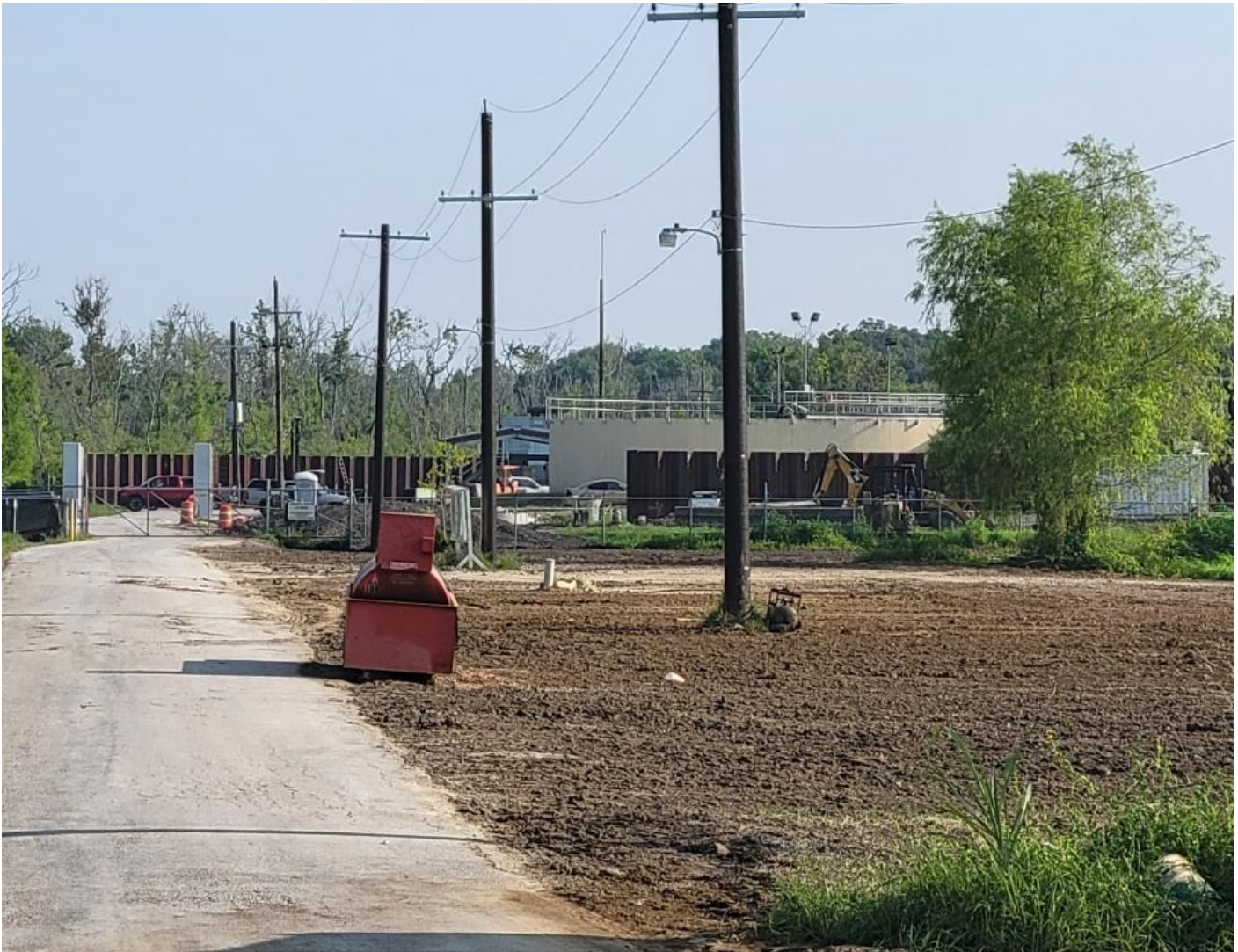
SHEET PILING ALONG THE FRONT OF THE WW TREATMENT PLANT
