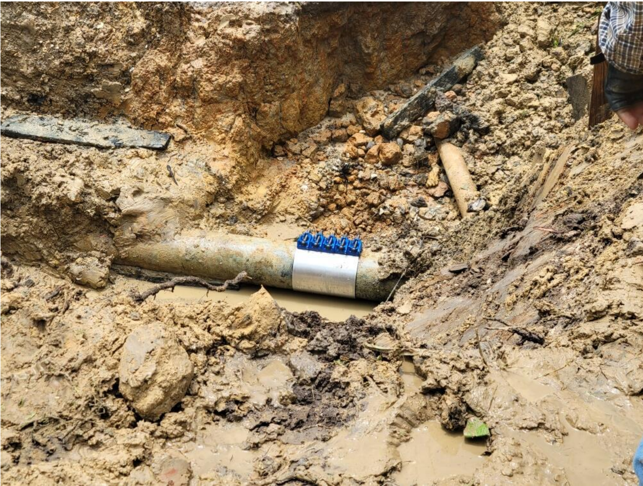
Repaired water leak with a 8" clamp
