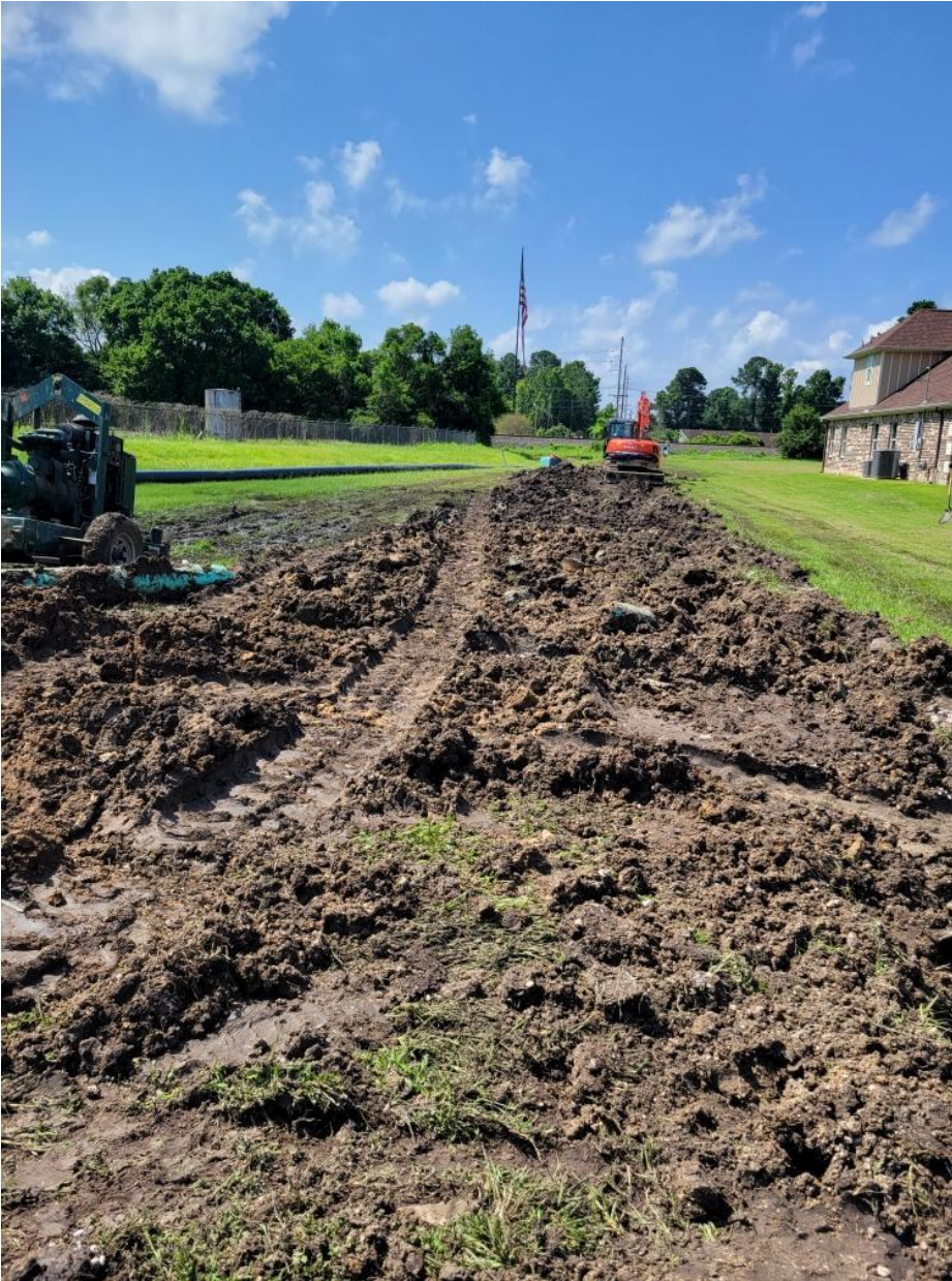
INSTALLATION OF 16" SEWER LINE ON BEAUMONT ST
