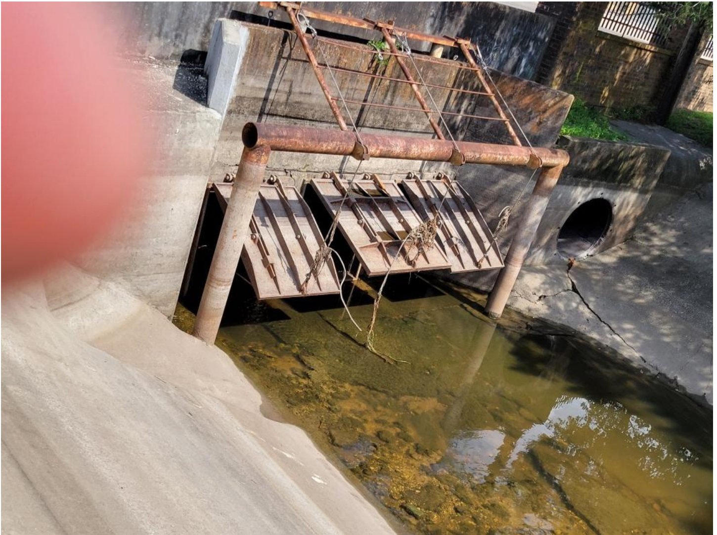
Main B with the flap gates opened on July 23, 2021
